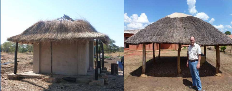
Innovative in our project is the introduction of *ShadeBots™* to stand alongside CoolBots™ and in providing shade above the CoolBot™ to reduce heat-load on structure
