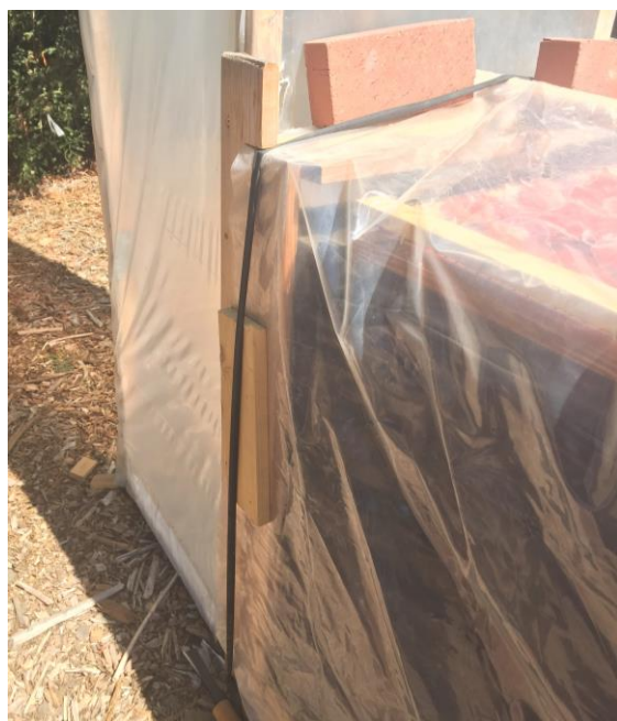
Figure 5 (left). A bicycle tire inner tube and bricks used to seal the table and chimney.
